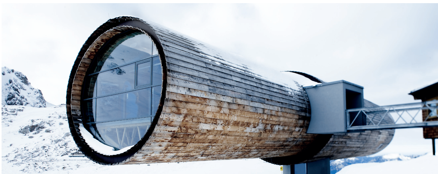
Mountain station Karwendel, Mittenwald Germany
